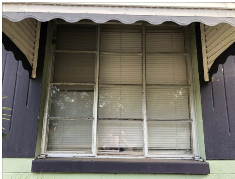
Figure 2: Photograph of historic window to be replaced.
